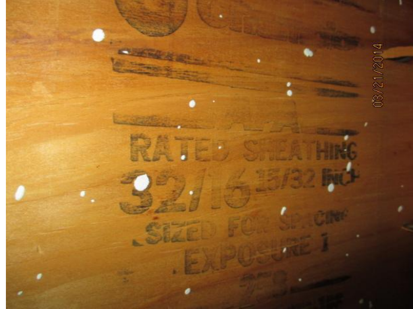
15/32" Deck Thickness Confirmed
