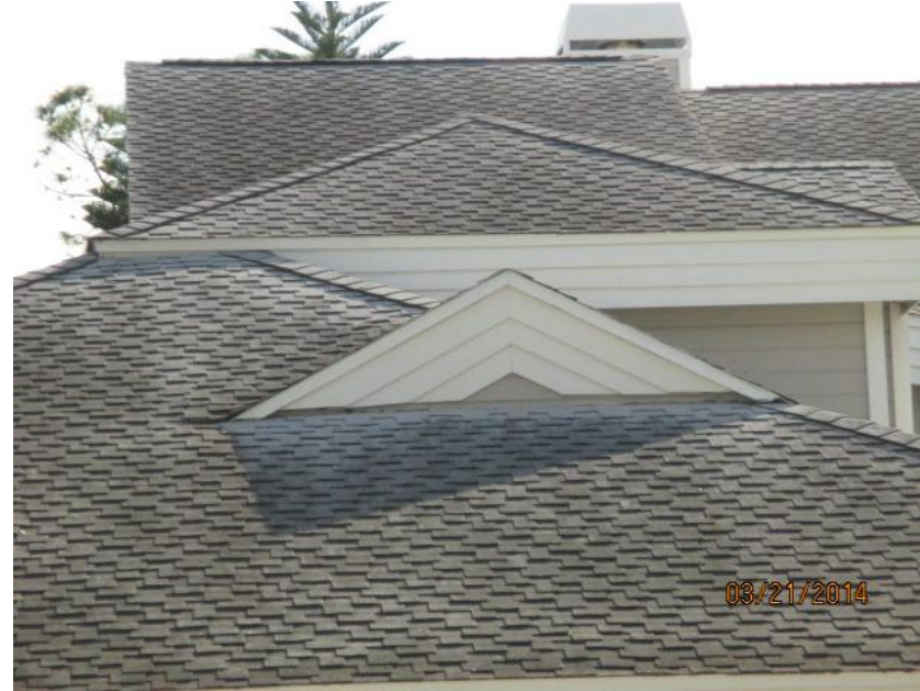
Asphalt/Fiberglass Shingle Roof Covering
