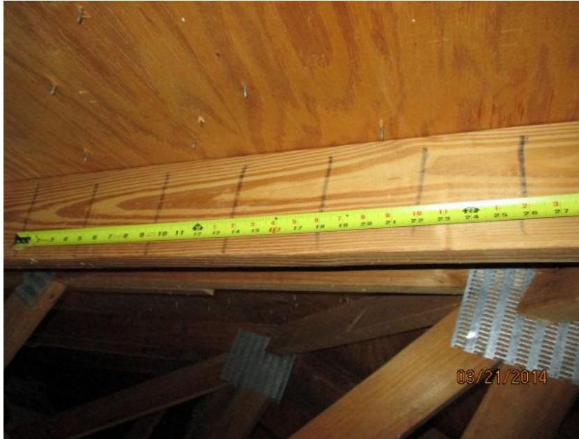
7d Nails Spaced 6" Along the Edge
