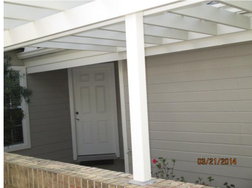
Unprotected Solid Entry Door
