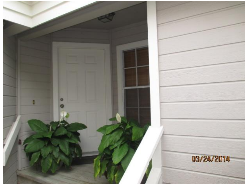
Unprotected Solid Entry Door
