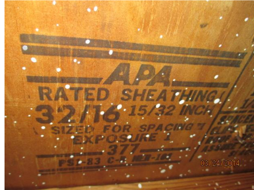
15/32" Deck Thickness Confirmed
