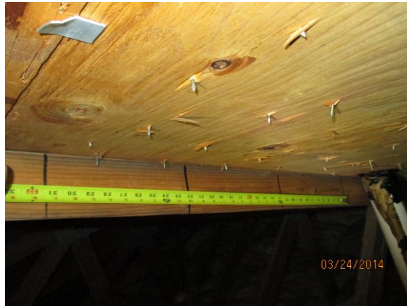
6d Nails Spaced 12" in the Field
