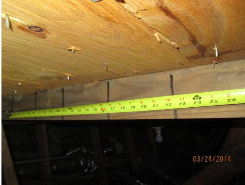
6d Nails Spaced 6" Along the Edge
