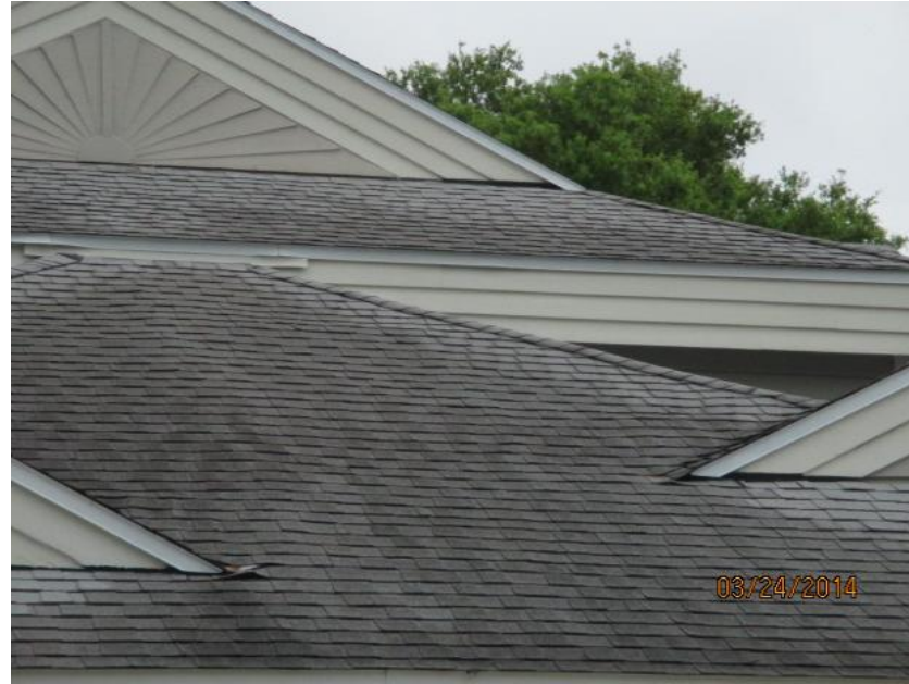
Asphalt/Fiberglass Shingle Roof Covering
