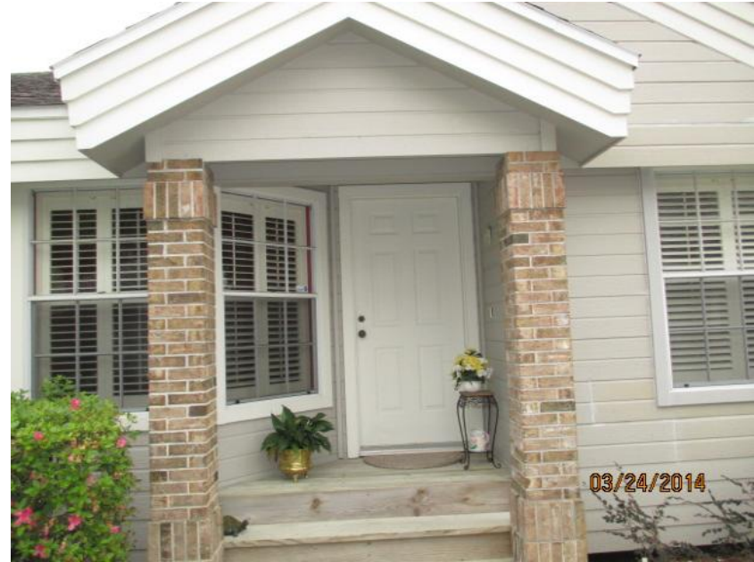
Unprotected Solid Entry Door
