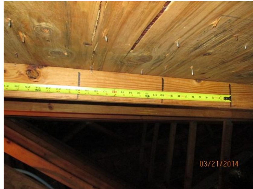
6d Nails Spaced 12" in the Field
