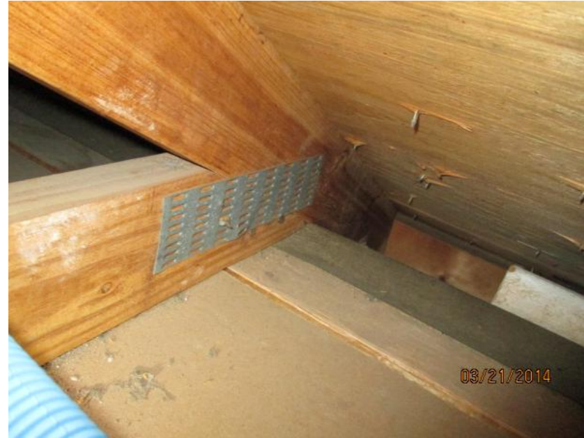
Clip with 3 nails on the front side and 0 nails on the opposing side
