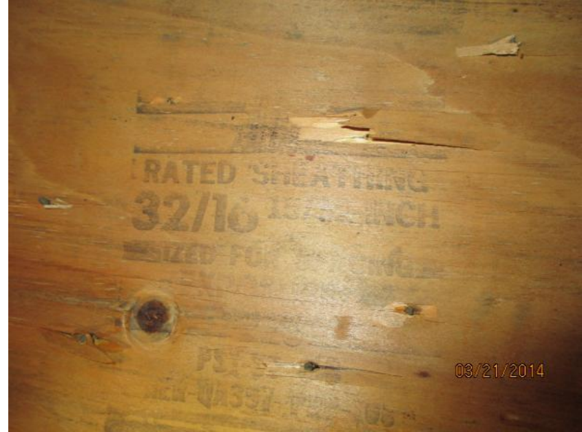
15/32" Deck Thickness Confirmed
