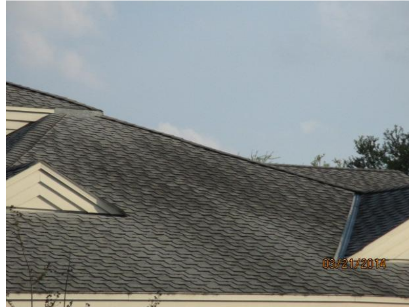
Asphalt/Fiberglass Shingle Roof Covering
