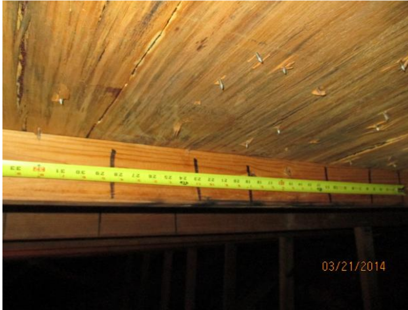
6d Nails Spaced 6" Along the Edge
