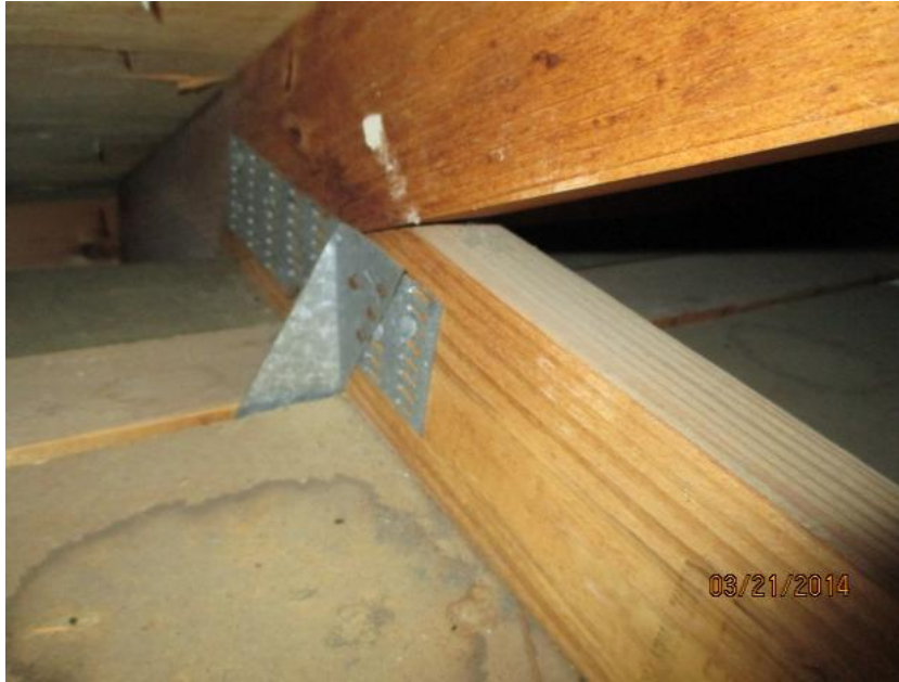
Clip with 3 nails on the front side and 0 nails on the opposing side
