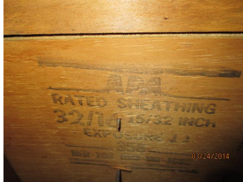
15/32" Deck Thickness Confirmed
