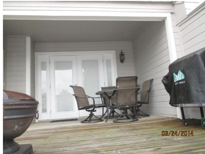
Unprotected Glazed Entry Doors
