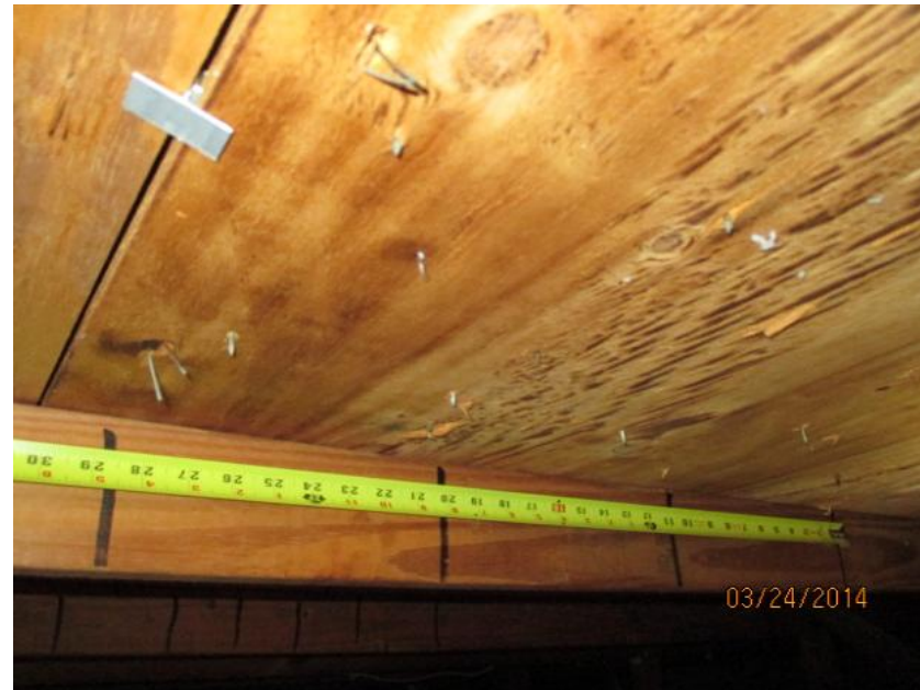
6d Nails Spaced 12" in the Field
