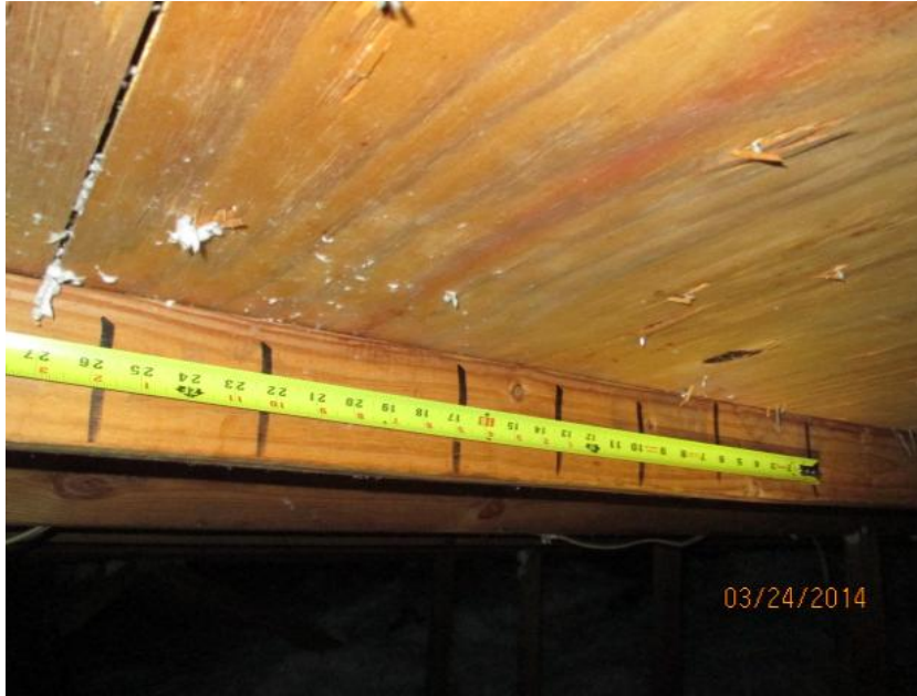
6d Nails Spaced 6" Along the Edge
