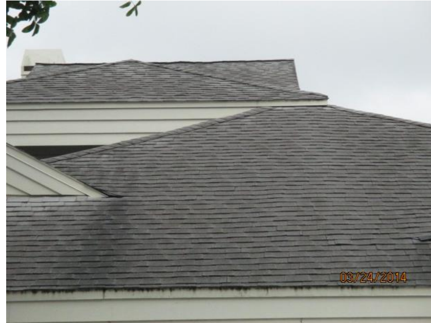
Asphalt/Fiberglass Shingle Roof Covering
