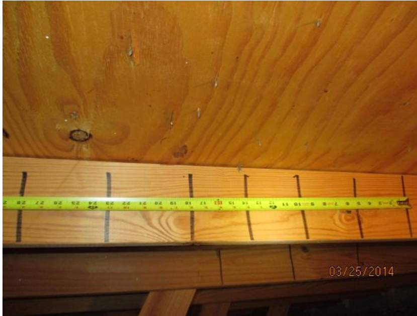
8d Nails Spaced 6" Along the Edge
