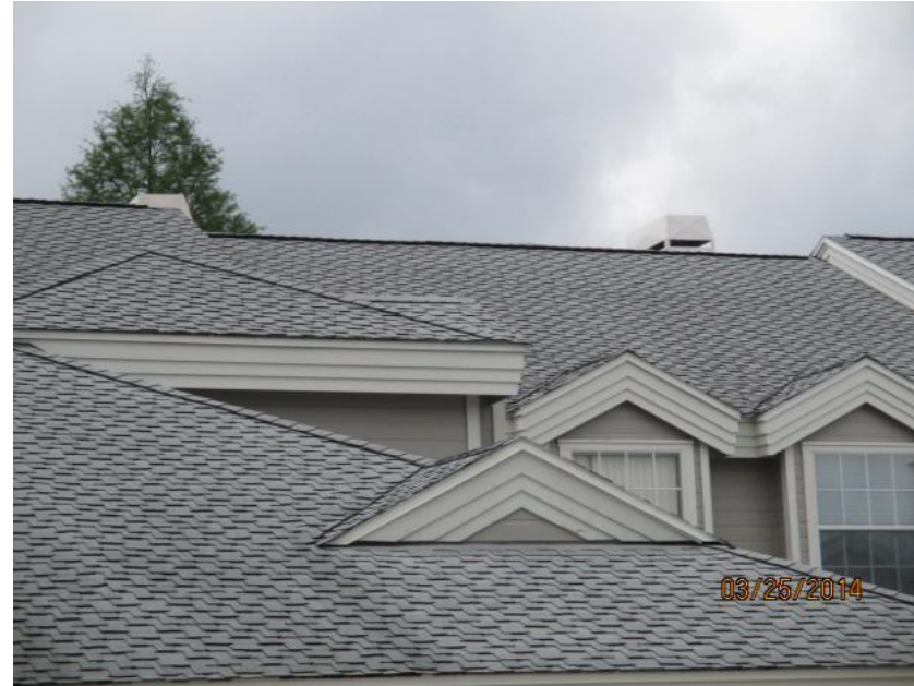
Asphalt/Fiberglass Shingle Roof Covering
