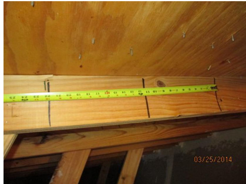
8d Nails Spaced 12" in the Field
