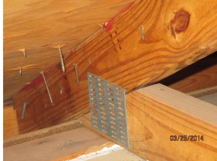
Clip with 4 nails on the front side and 0 nails on the opposing side
