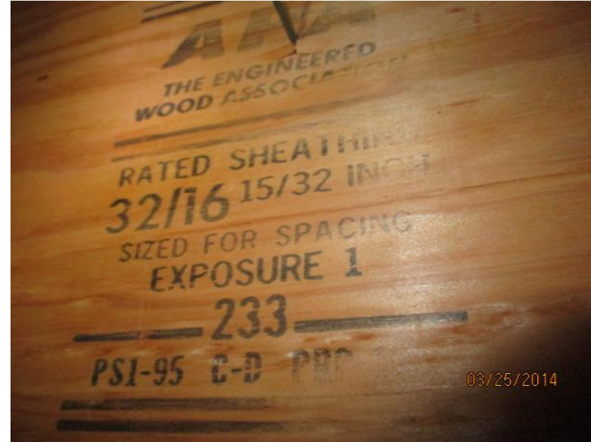
15/32" Deck Thickness Confirmed
