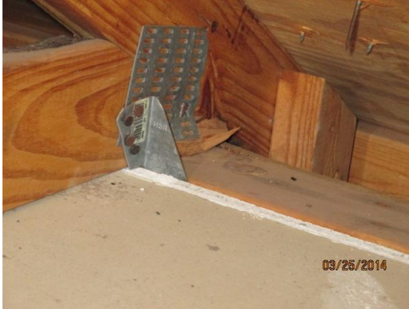
Clip with 4 nails on the front side and 0 nails on the opposing side
