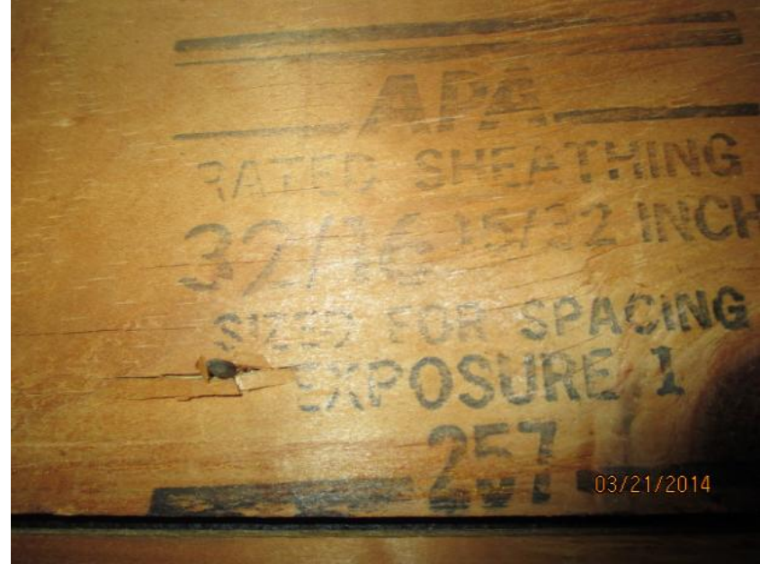
15/32" Deck Thickness Confirmed
