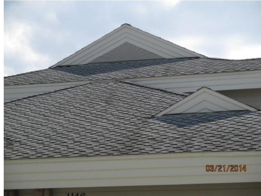
Asphalt/Fiberglass Shingle Roof Covering
