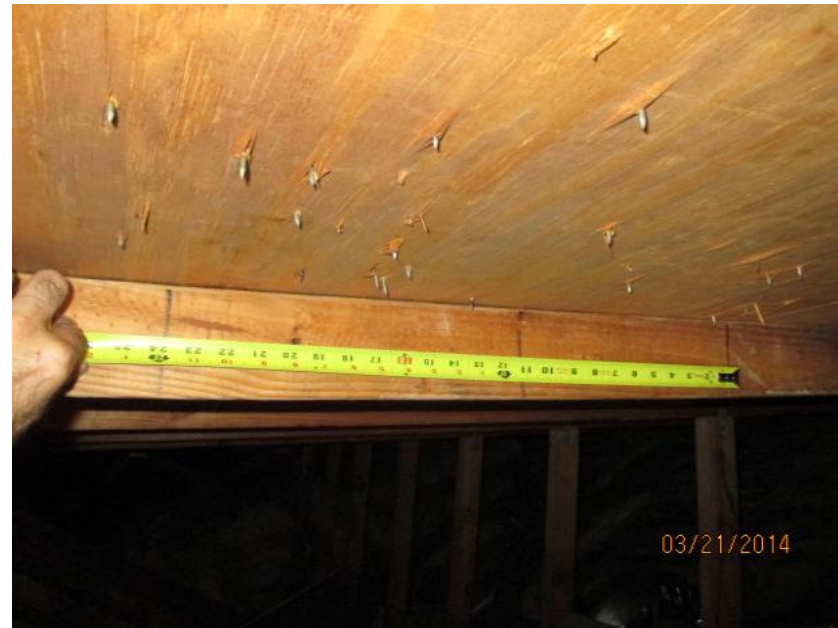
6d Nails Spaced 12" in the Field
