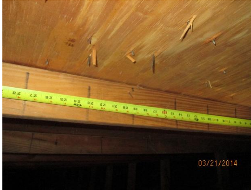
6d Nails Spaced 6" Along the Edge
