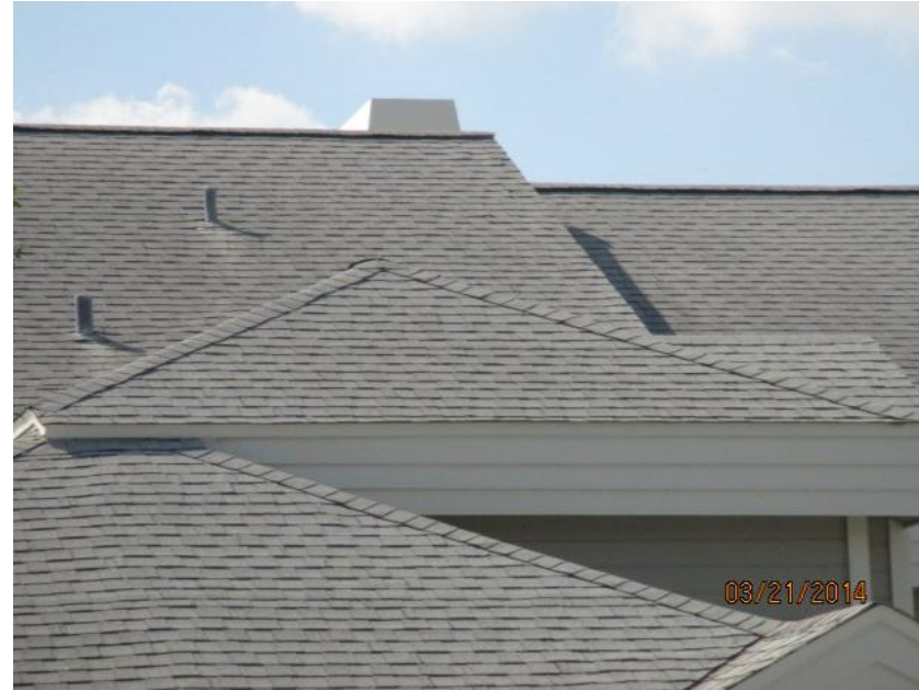
Asphalt/Fiberglass Shingle Roof Covering
