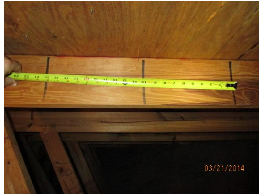
6d Nails Spaced 12" in the Field
