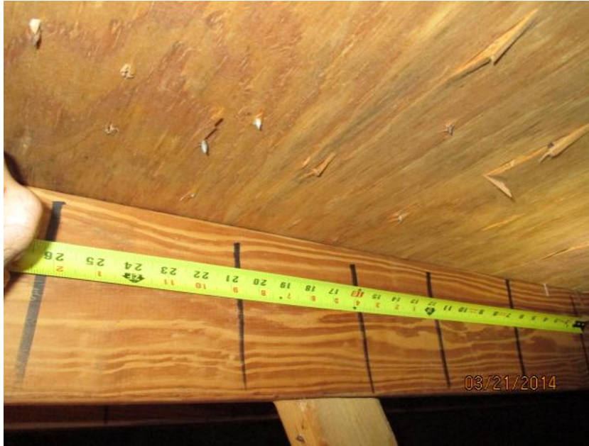
6d Nails Spaced 6" Along the Edge
