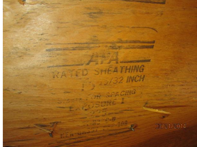
15/32" Deck Thickness Confirmed
