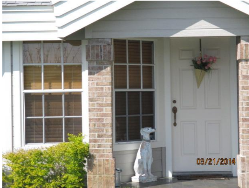
Unprotected Solid Entry Door
