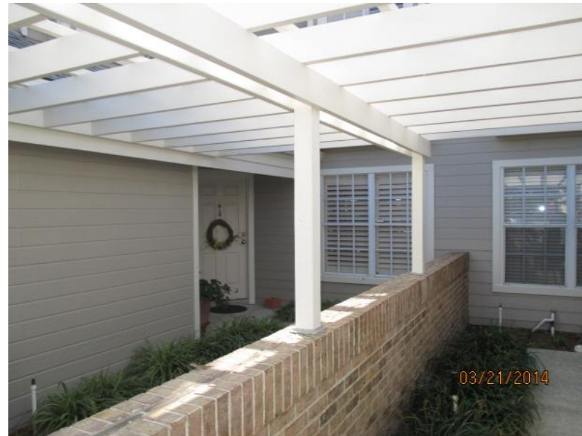
Unprotected Solid Entry Door
